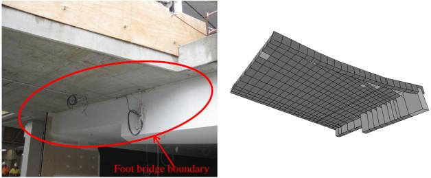
Figure 7. View at the boundary and the extruded view of the updated SAP model
